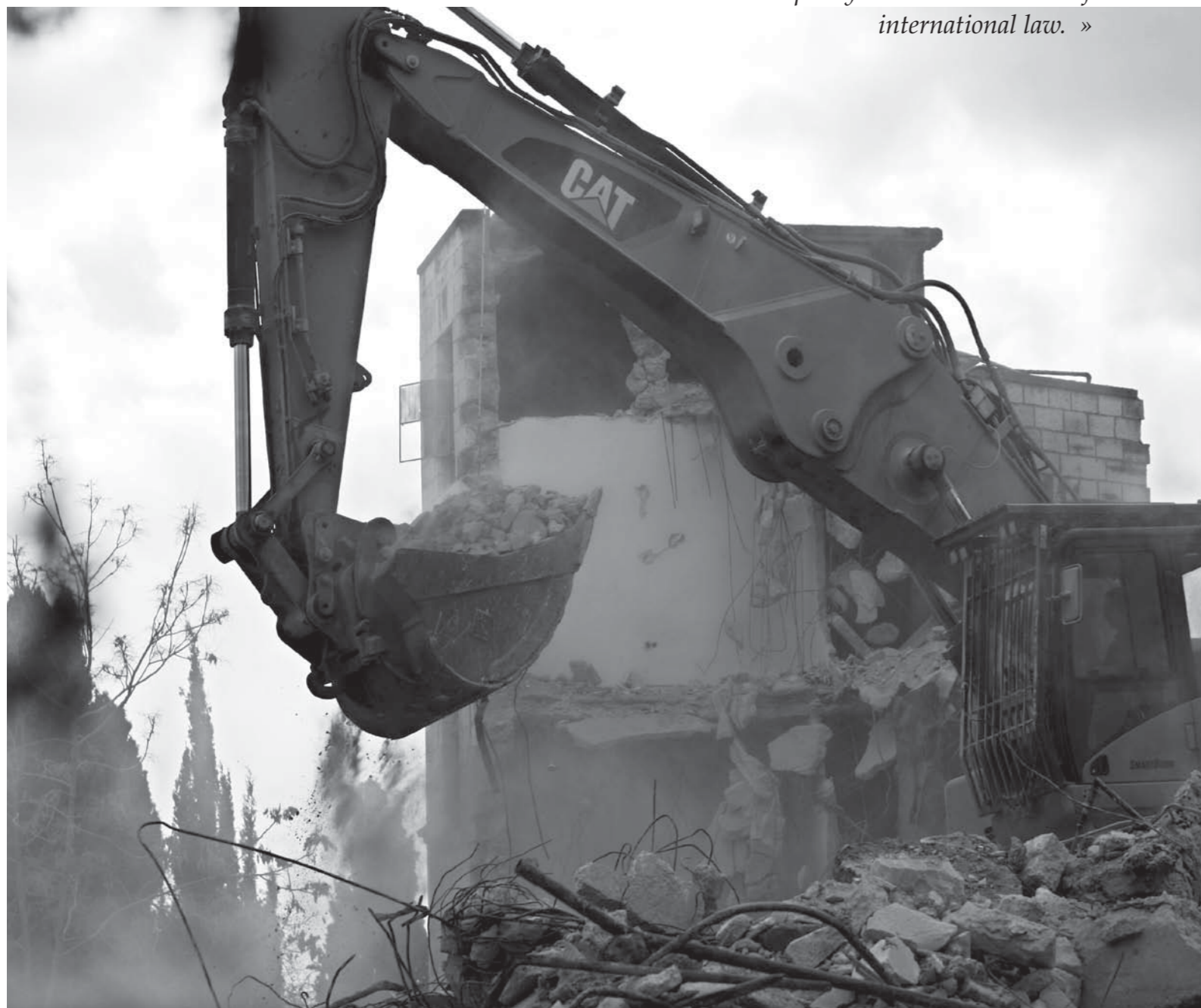
The demolition of the Shepherd Hotel in Sheikh Jarrah, East Jerusalem, 9 January 2011 © Atef Safadi
